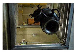
Fig 5. Pump being lowered into the shaft
